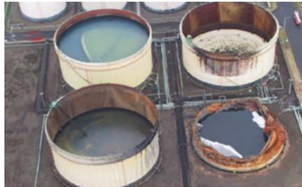
**Fig.4. Floating-roof damage.**
