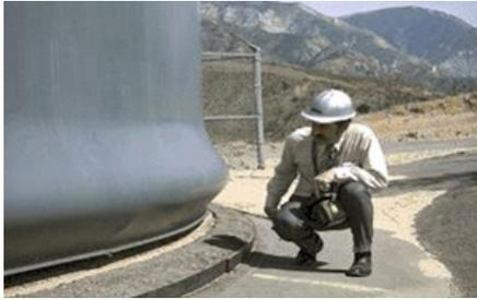
**Fig.2. Shell elephant's foot buckling or elastic-plastic buckling.**
