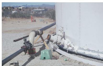
**Fig.5. Detachment of the pipe due to sliding and shell buckling.**
