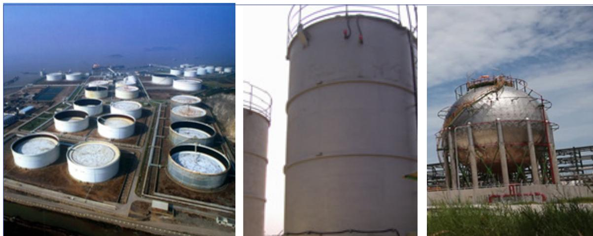
**Fig.1. Typical tanks in an oil and gas industrial storage facilities (l-r): (a) broad tank, (b) slender tank, and (c) spherical LNG tank.**
